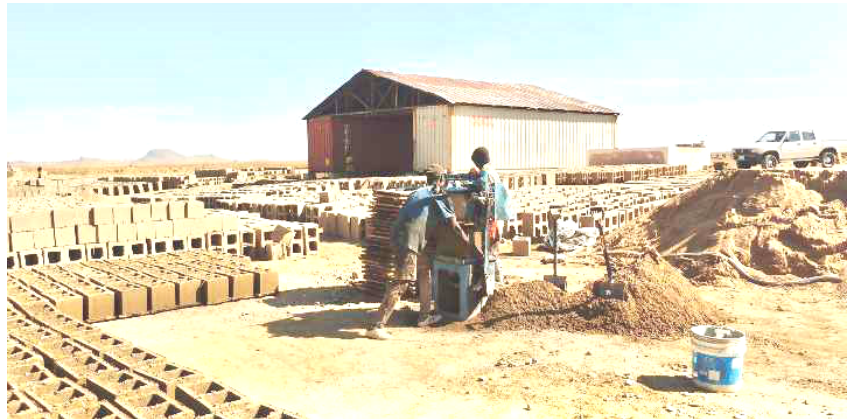
Block manufacturing on site
